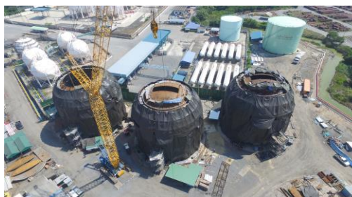
WP BangPa-kong LPG Terminal Phase 3(EPC)
