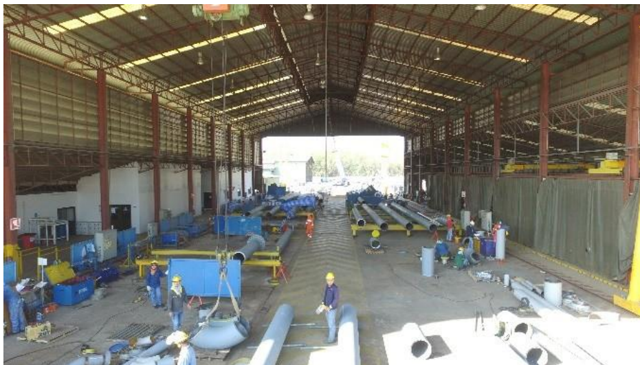
Steel Structure Fabrication
