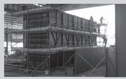
Heat exchange pipe fabrication and assembly
