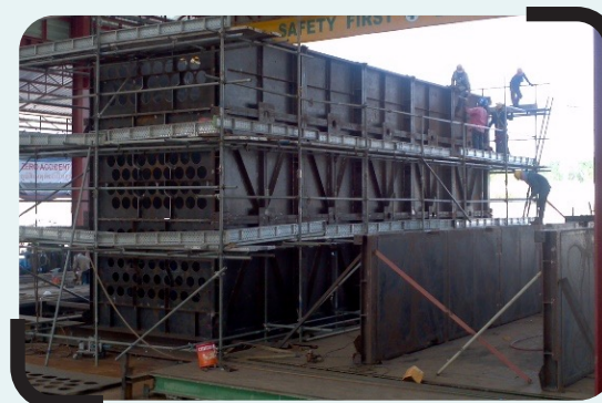
Heat exchange pipe fabrication and assembly
