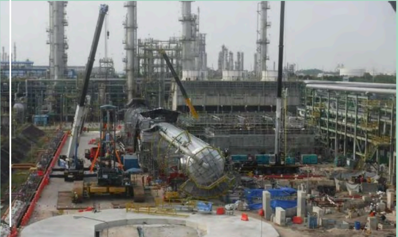
PTT GC OMP Project (General Construction)
