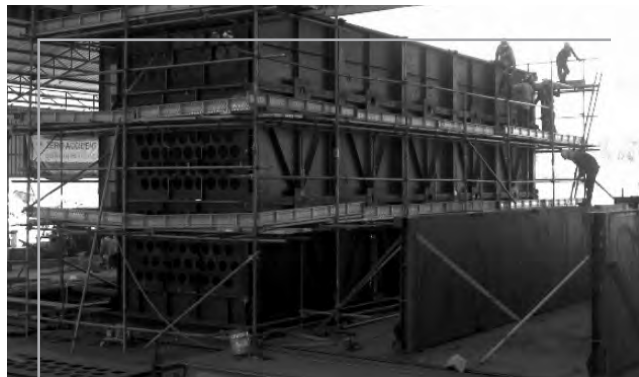
Heat exchange pipe fabrication and assembly
