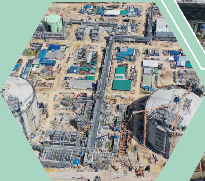
PTTLNG Receiving Terminal Nongfab Project (Civil)
