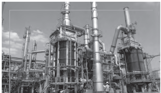
Project: BCP Continuous Catalyst Regeneration (CCR) and Hydrocracker Unit (HCU) Civil
