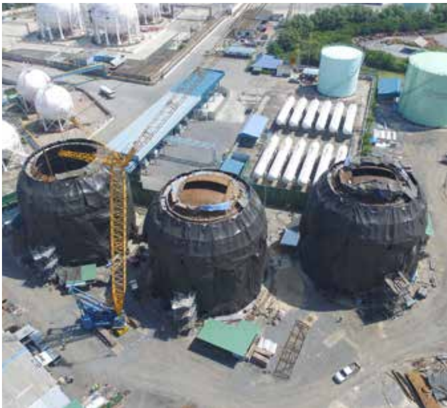
WP BangPa-kong LPG Terminal Phase 3 (EPC)
