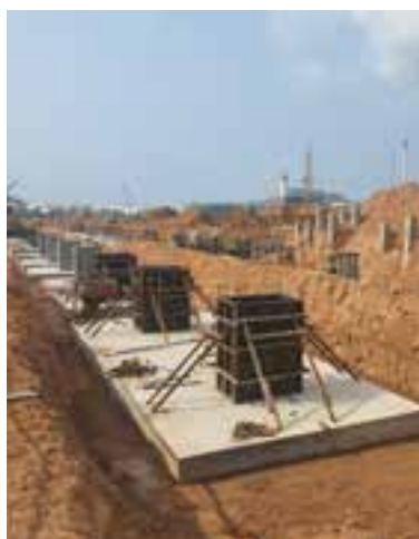
Thaioil Clean Fuel (Civil)
