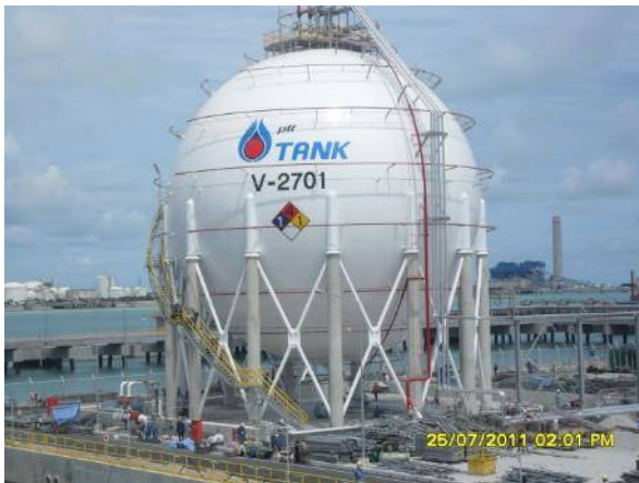
PTT Tank Terminal PP Tank
